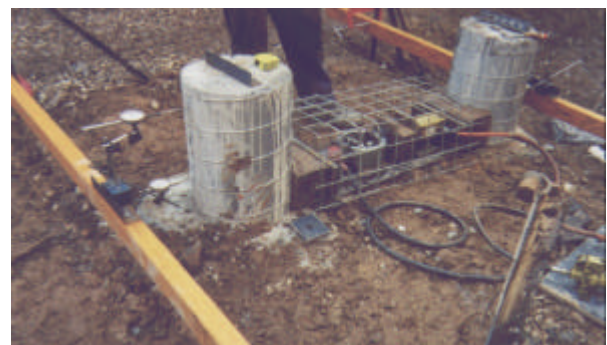
Figure 3. Lateral load test arrangement
