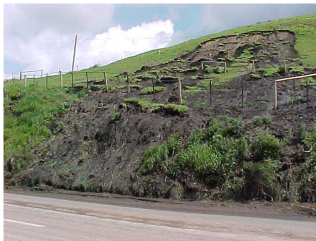
Figure 3: Two adjacent landslides that impacted on the Great Ocean Road, October 2000.
