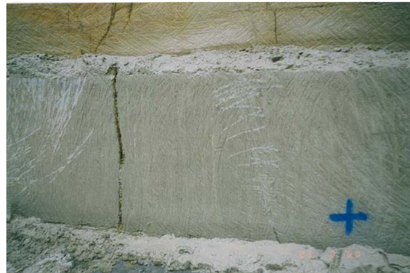
Figure 9: Close up view of open joint terminating on laminite/shale bedding seam at base of photo.
