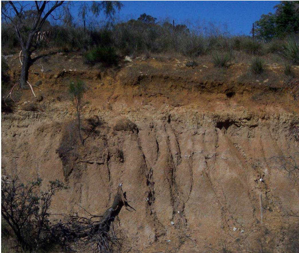
Figure 13: Hard bed - indurated calcareous mudstone in the upper third of this section in the Guildford Formation, in the railway cutting, Hallatt Gardens, Upper Swan River.
