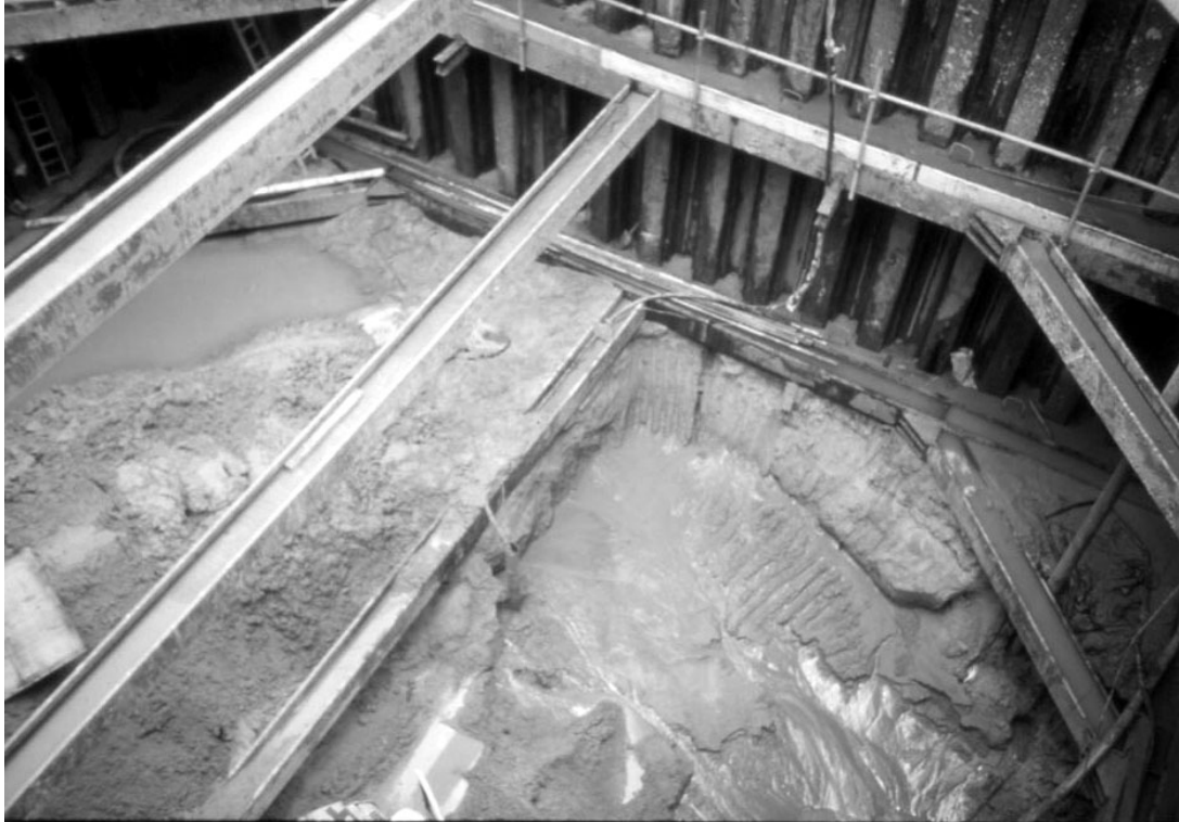
Figure 7: Organic channel sands, in air shaft for Bermondsey Station, Jubilee Line Extension project (Upper Mottled Beds, Reading Formation).
