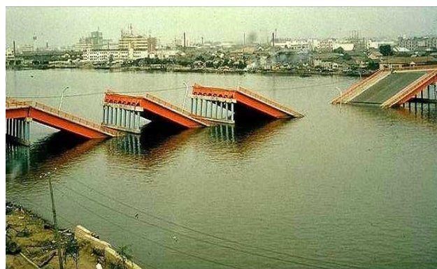
Figure 2: Bridge failure by liquefaction in the 1964 Niigata earthquake (photo courtesy NISEE)
