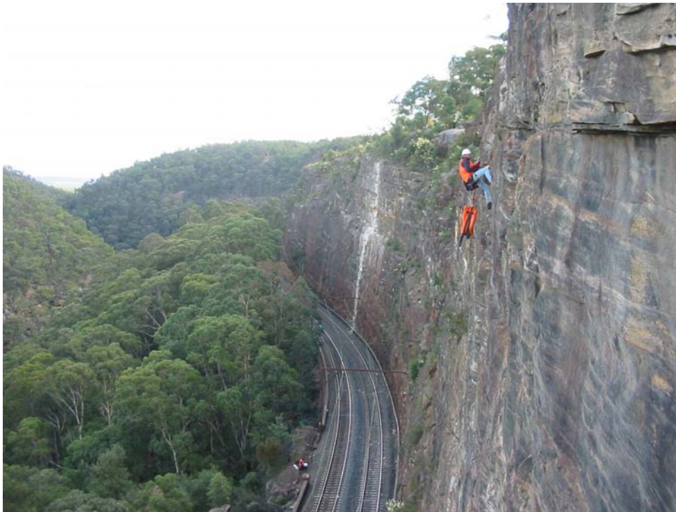
Figure 1: Engineering Geologist assessing slope hazards on the Eastern Cut.
