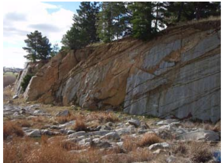
Figure 5 spillway excavation in variably weathered granite (F5)
