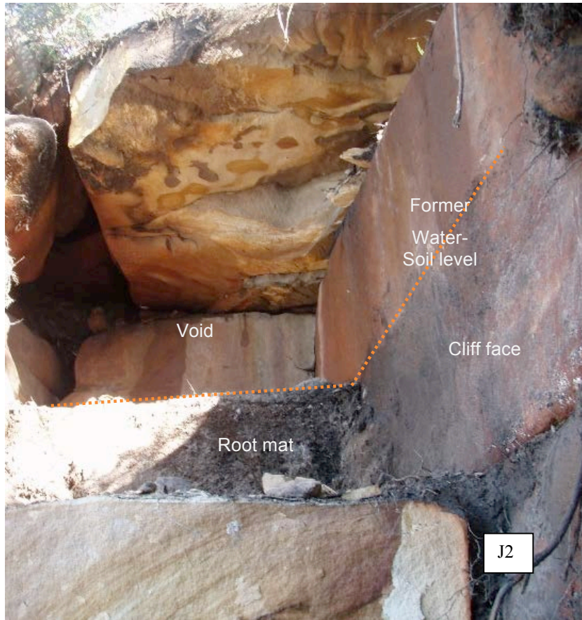
Figure 6: Photo showing open void that existed at the rear of B3 when it was in situ .
