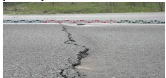
Pic. 2-1. A linear-type discontinuous surface deformation (Grygierek 2010)
