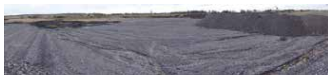
Figure 12. Progress of capping of TSF1 as at 25 June 2015, showing the initial 1 m thick layer and the follow-up 2 to 3 m thick layer of coarse reject.
