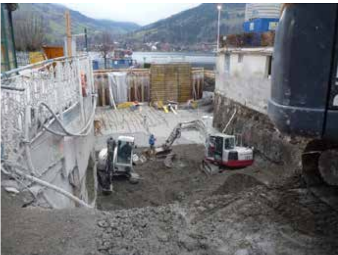
Figure 9. Picture of excavation and soilcrete columns
