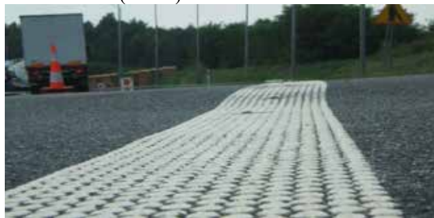
Pic. 7-4. Deformation of the northern roadway of A4 motorway - 5 August 2010 (Grygierek at al. 2015 )
