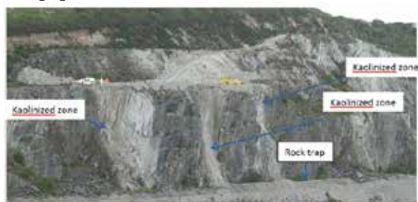
Figure 1. Photograph of a section of historical bench face (striking N-S) with several sub-vertical kaolinized zones, found within poorly kaolinized rock. Discontinuities sets of high angle joints striking sub parallel to the face subject to possible toppling failure.
