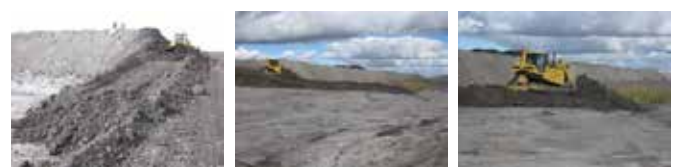
Figure 9. Early pushing of a capping of coarse reject over old bow-wave of surface TSF.
