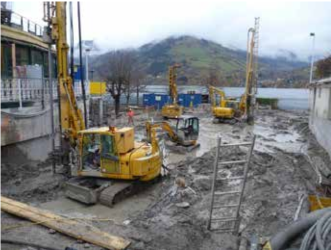
Figure 8. Picture of Jet-Grouting-Works
