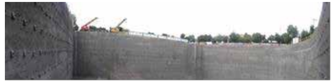
Fig. 1 A view of walls stabilized by nailing
